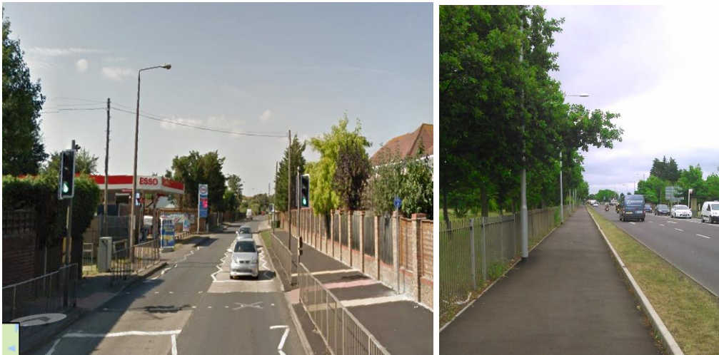
Figure 4.1: Shared footways on Somnes Avenue and Canvey Road
